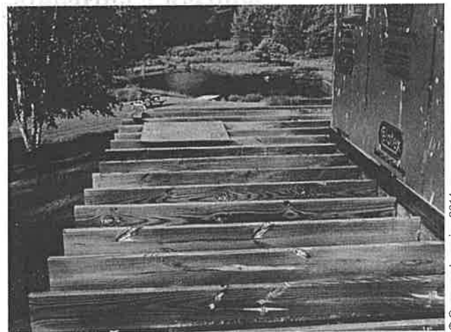
FIGURE 1-6 Joists set for a deck by carpenters.
