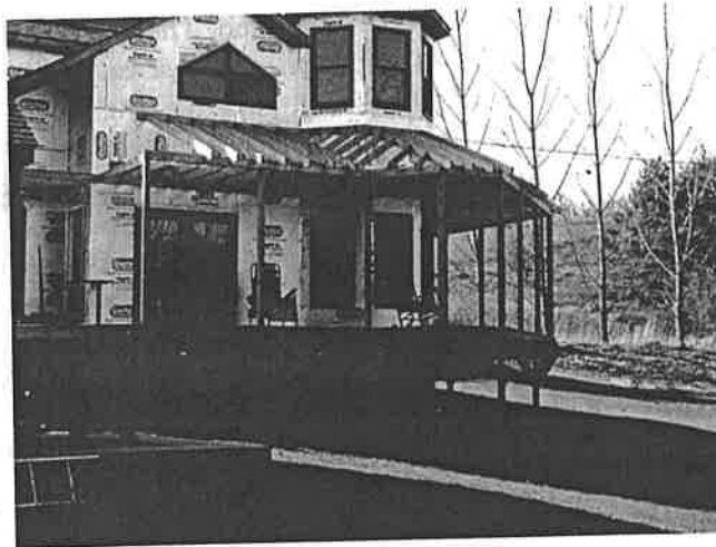
FIGURE 1-8 Porch roof framed by carpenters.
